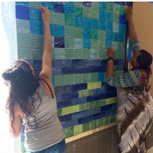
MudGirls work on the fireplace in the Stockton residential building
